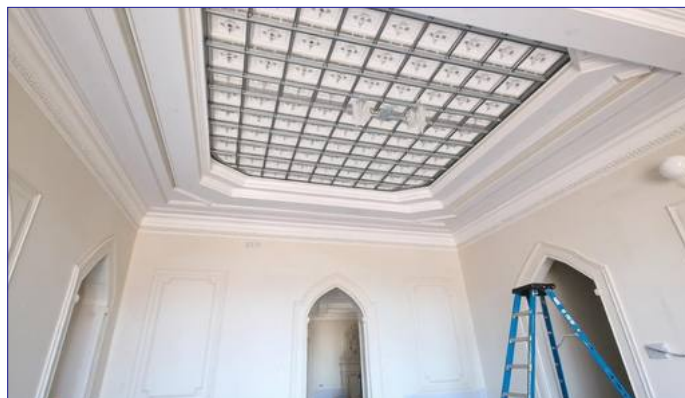
DURING — WORKS IN PROGRESS
