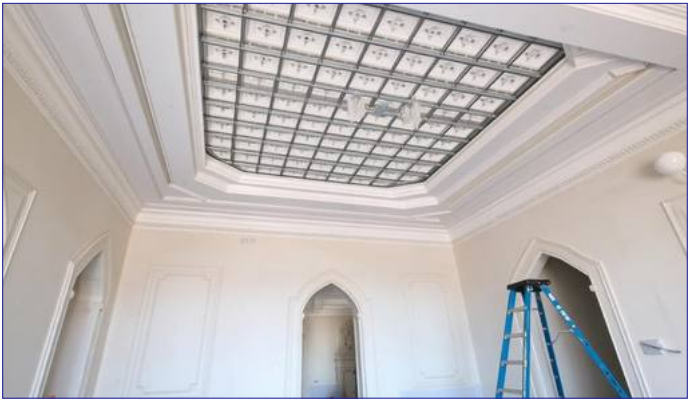
DURING — WORKS IN PROGRESS
