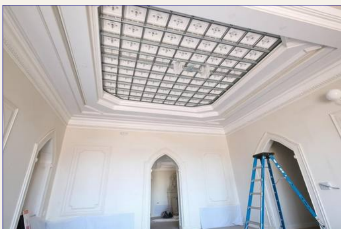
STAGE 03 — CEILINGS & PLASTER
