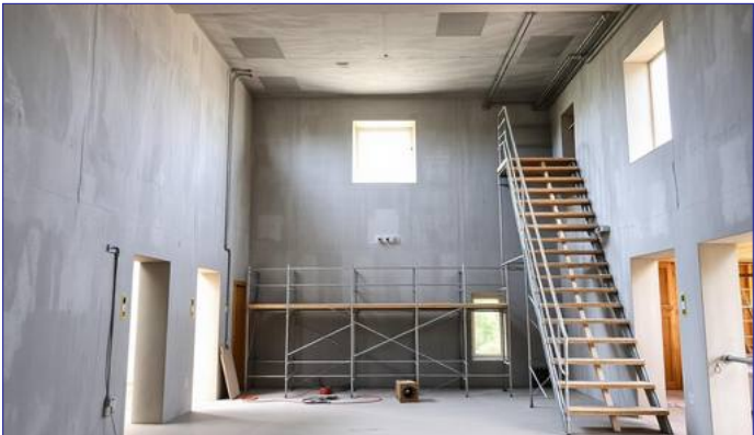
DURING – WORKS IN PROGRESS
