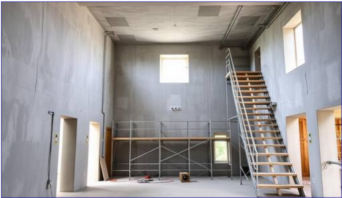
DURING — WORKS IN PROGRESS
