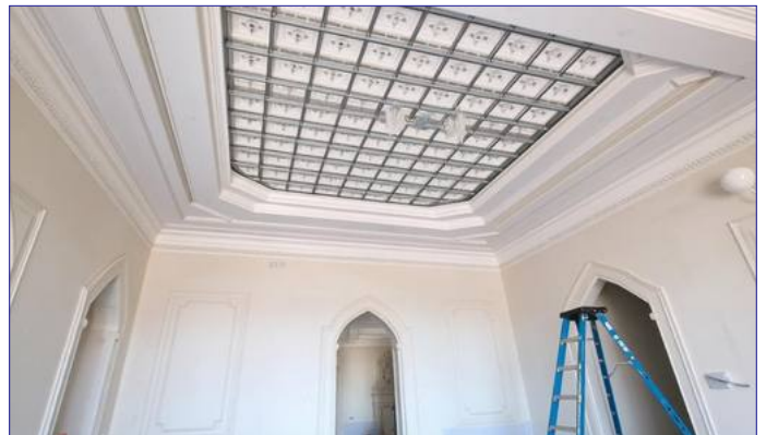
DURING — WORKS IN PROGRESS
