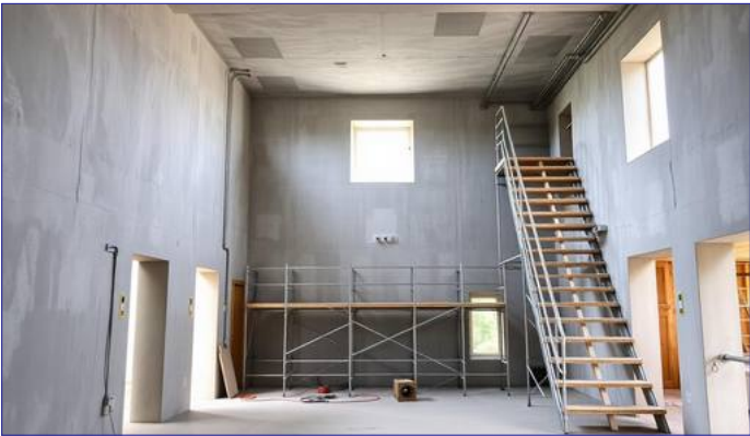
BEFORE — EXISTING CONDITION PROGRESS IMAGES SHOWN ARE REPRESENTATIVE OF THE WORKS CARRIED OUT.
